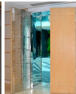
Wood door with laminated wood veneer on one side and stainless steel strips on the other side to give 2 different ambiance matching the architectural design
